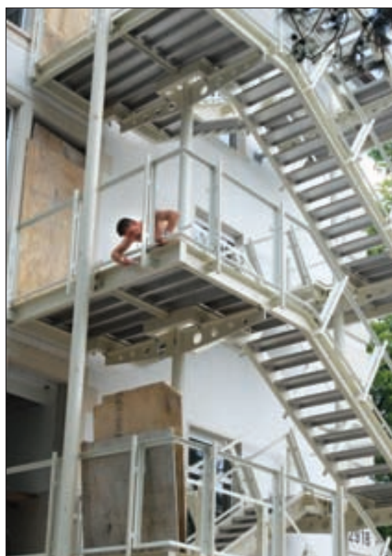
[Above] A worker prepares a crane to move dirt from the area in front of Patch High School, near a recently-removed tree stump. The area was renovated to make room for a new emergency evacuation route, which includes an outdoor elevator. [Left] A worker paints part of the newly-installed fire escape at Böblingen Elementary/Middle School on Panzer Kaserne. The fire escape project's final phase was completed this summer.
